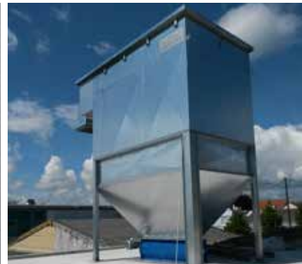
Extraction unit MMJet 300 with rotary valve
